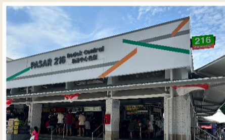
Kampong Chai Chee: Repairs & Redecoration at Pasar 216 Market
