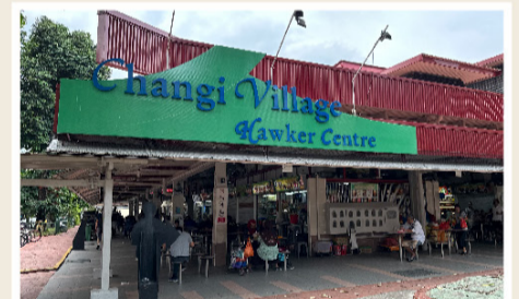
Siglap: Repairs & Redecoration of Changi Village Hawker Centre
