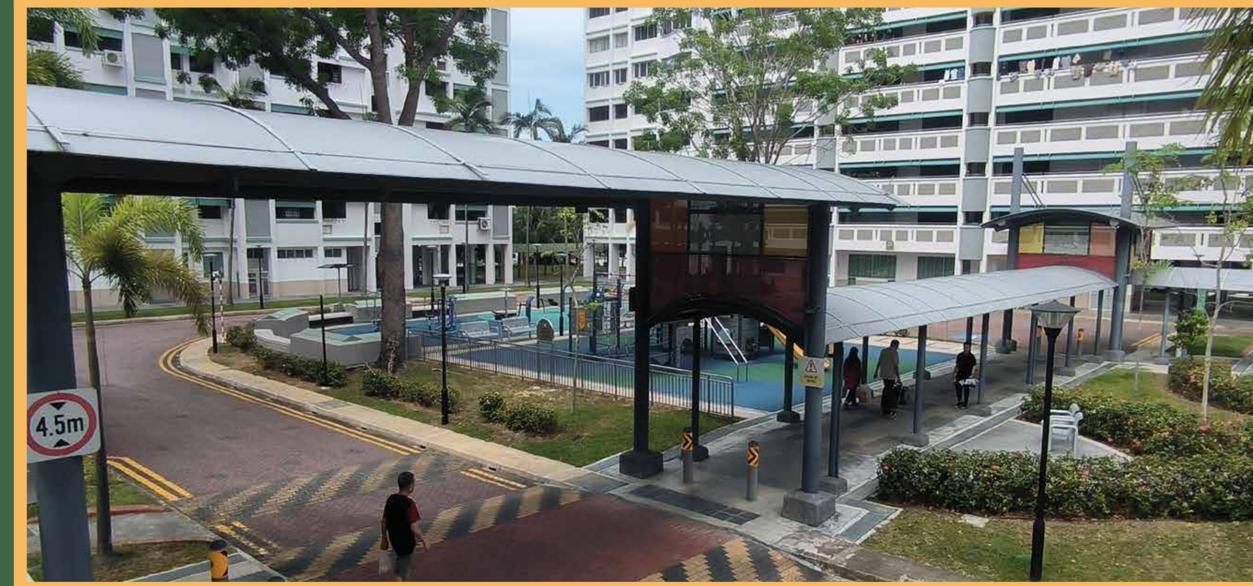
Convenient connectors and sheltered linkways throughout Changi Simei estates
