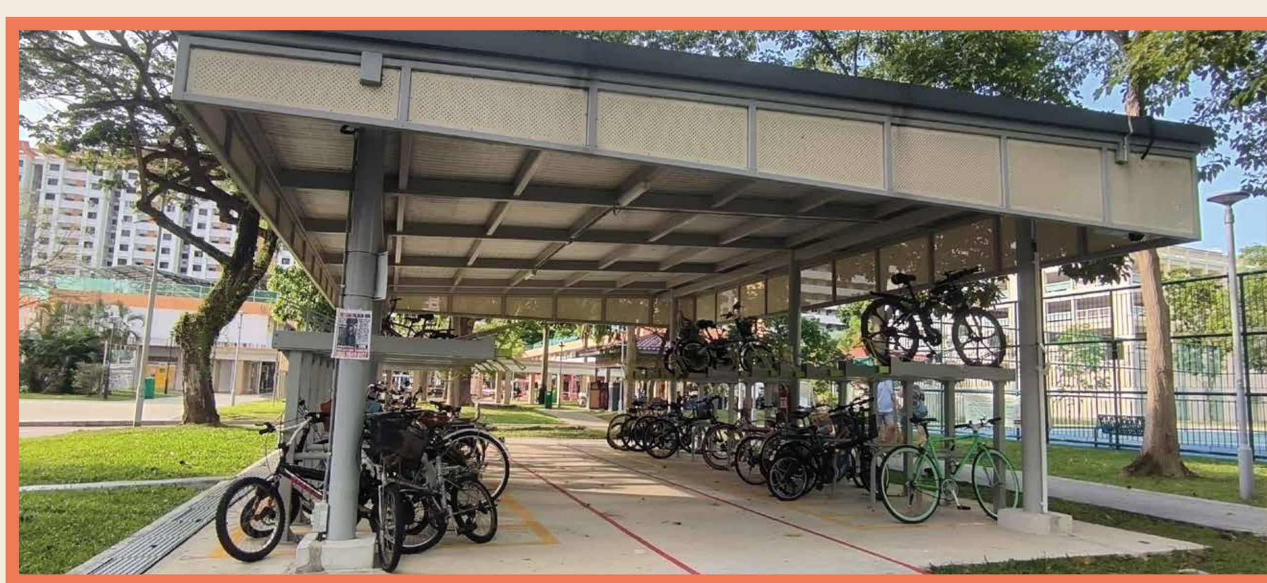
Double tiered bicycle racks at Blk 56 and Bedok South Road to promote active mobility
