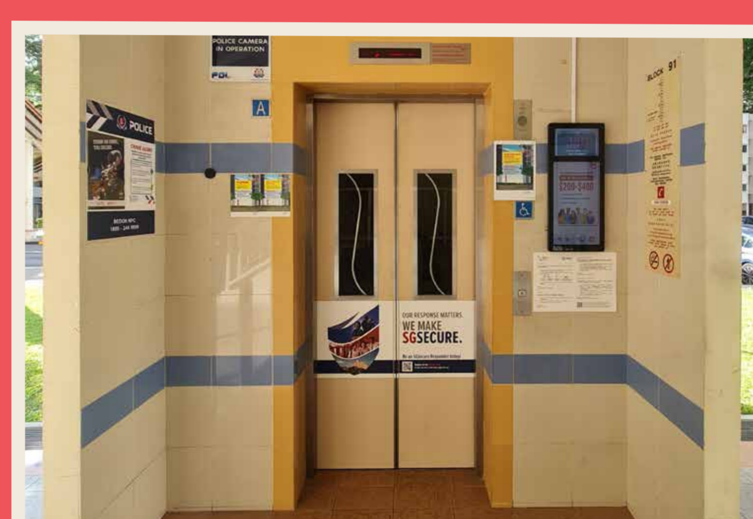
Upgrading older lifts to meet new safety standards at Blk 90 to 94B
