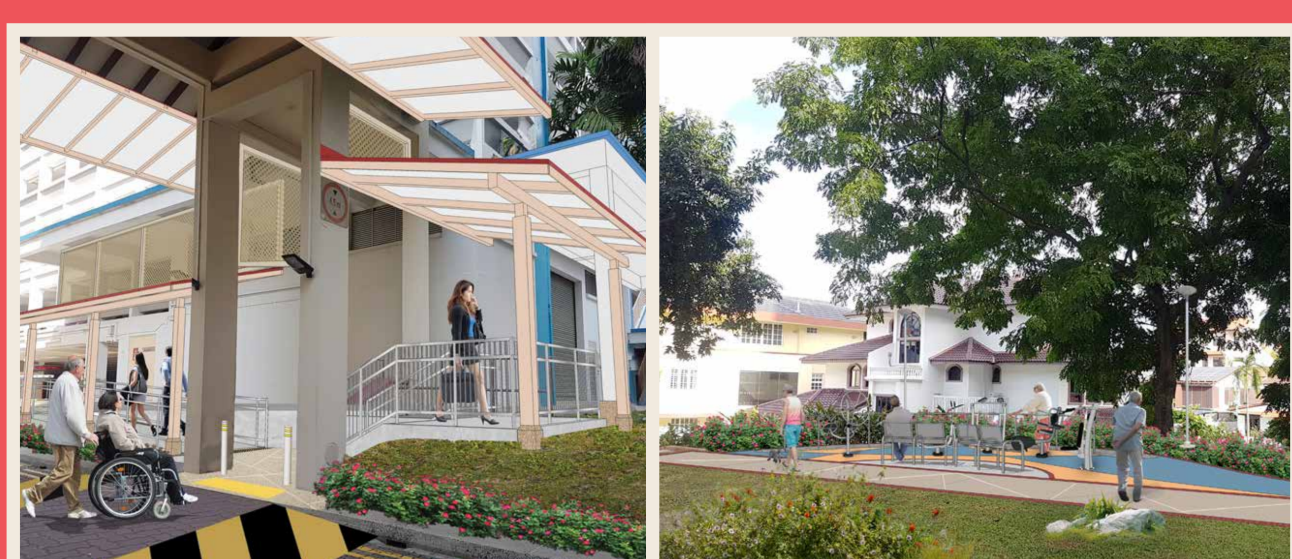
Upcoming rejuvenation of living environment through Neighbourhood Renewal Programme at Blk 94B/C/D/E Bedok North Ave 4
