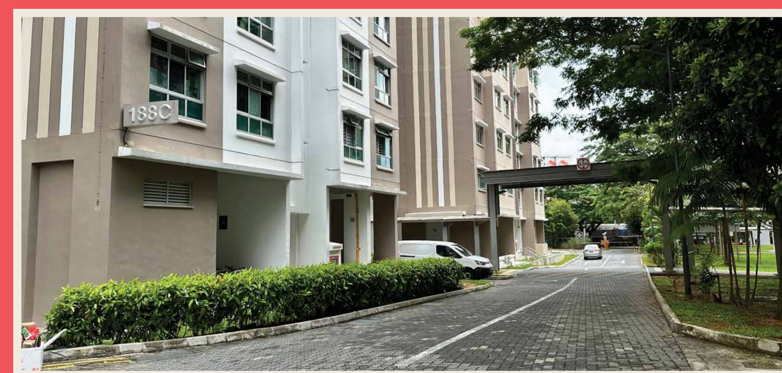
A safer environment with widened walking space at Blk 188C
