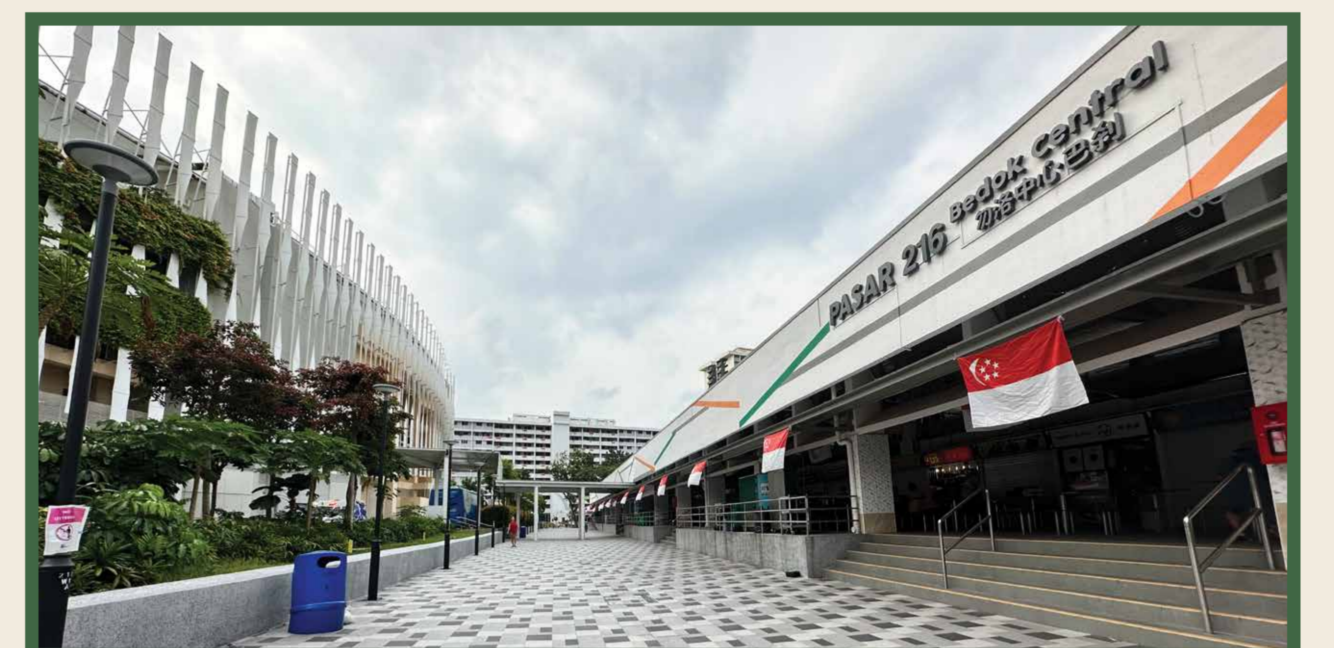
Wider walkway for the safety of pedestrians and cyclists between Blk 216 and Heartbeat
