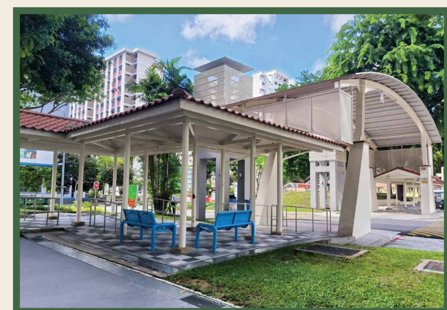
All weather protection from Blk 401 to 406
