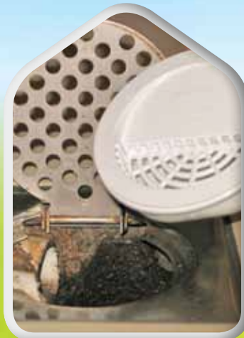
Install anti-mosquito valves, to cover the rarely used gully traps
