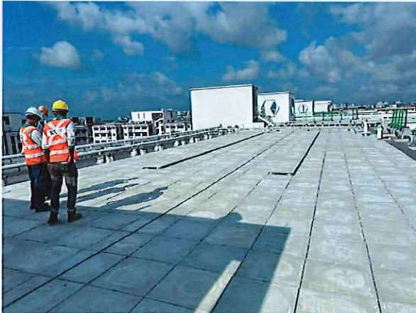
Re-Roofing (Changi Simei) 33 blocks @ Simei Street 1 & 5
